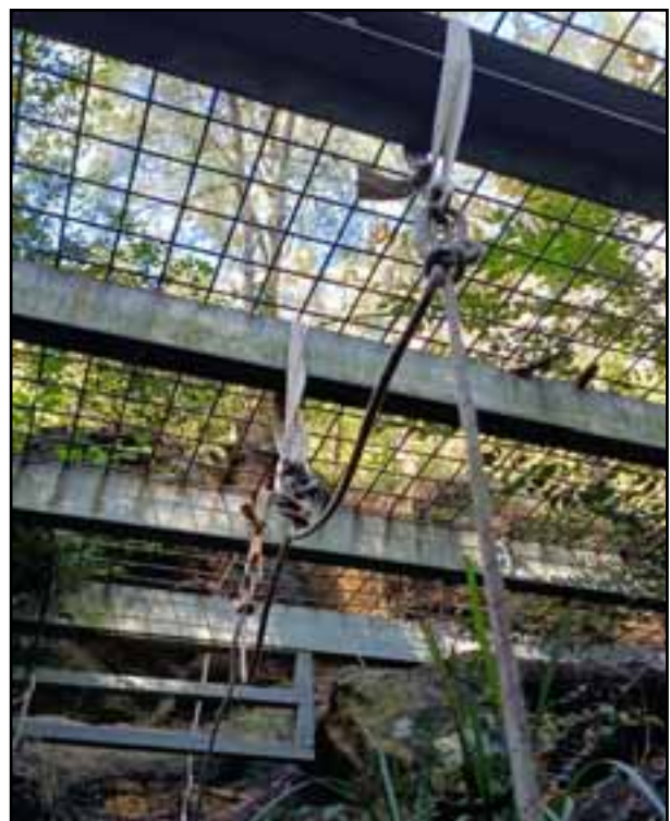
Photo 6: The rigging from below. Photo: Chris Curtis.
