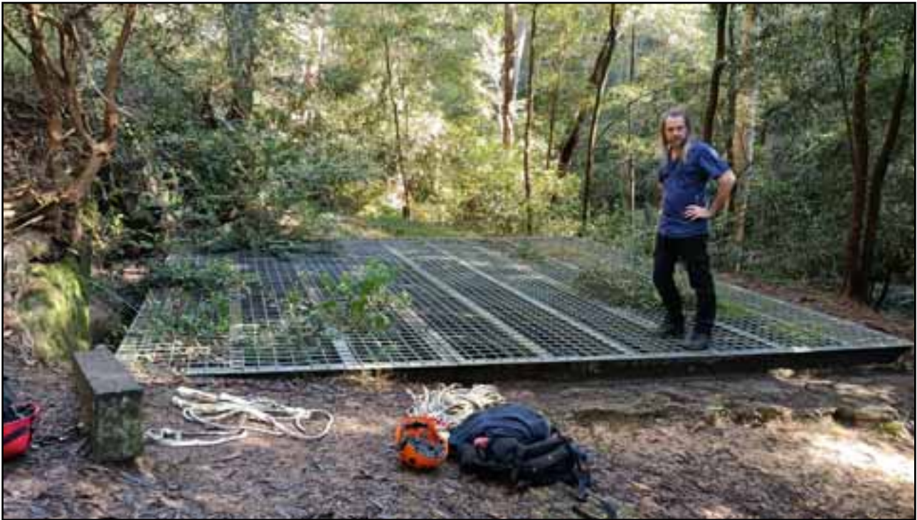
Photo 3: The large steel mesh covering of the Knapsack Creek Hole. Photo: Chris Curtis.
